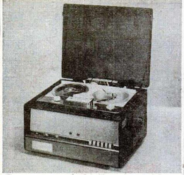
Here is the new portable version of the Bell & Howell Miracle 2000 tape recorder. Retailing at \$299.95, the unit features three separate motors, drop-in threading, dual-speed operation and a program indicator, which quickly locates each recording on a tape. Realistic sound reproductionunusual in a portable model—is achieved by the placement of four speakers two eight-inch woofers (one on each side) and two electrostatic tweeters in front.
