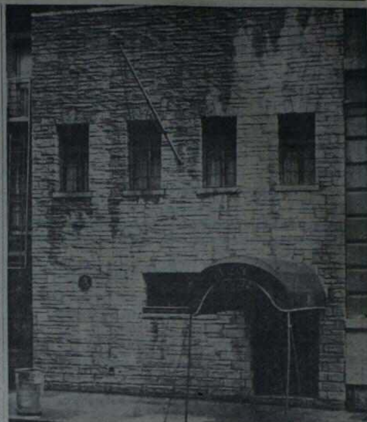
NEW HOME of the National Showmen's Association will be this two-story building constructed by the Friars' Club in 1950. Located between Sixth and Seventh avenues on 56th Street, New York, it contains large assembly rooms, offices, air-conditioning thruout, kitchen, lavatories on each floor, and cloak and storage rooms. Negotiations for its purchase have been proceeding for many months and a final meeting, at which the closing will be accomplished, has been set for this week. It will be the fourth meeting place of the NSA, which has been seeking to buy a permanent home for some time.
