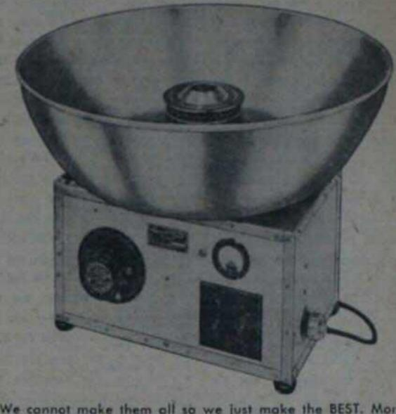
We cannot make them all so we just make the BEST. More than 50 years' experience. OUR PERFECTION is precision built, direct drive, built-in rheastat, valt meter. Fuse black and fuses-all aluminum housing no vibration, rubber mountings, all parts easily accessible. Each machine sugar tested before packing to be sure of 100% perfection, and guaranteed to be absolutely mechanically perfect.
