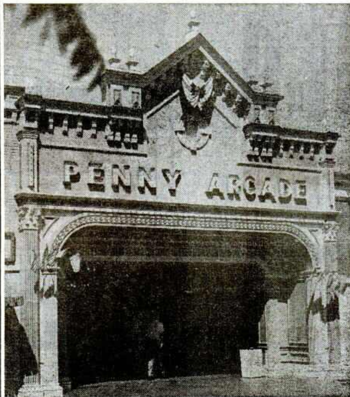
The Penny Arcade, located on the turn-of-the-century Main Street at Disneyland, is one of the top crowd pleasers at Anaheim. Esmeralda, a fortune-telling machine, heads the center line of antique games.
