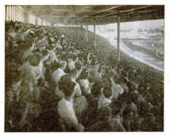
Relatively few column supports give patrons practically unobscured vision. Roof is hung on cantilever trasses supported by small number of steel columns.
