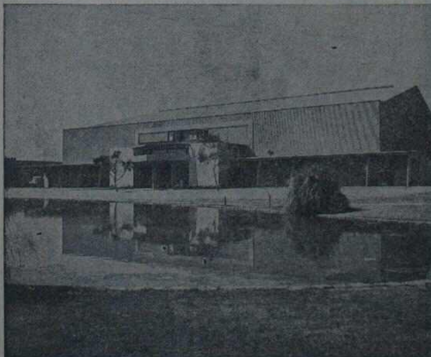
THE NATIONAL ORANGE SHOW is pushing its master development plan. Three major structures have been constructed since the war. At the top is the Industrial Building, first of these to go up; below it is Administration Building and at the bottom is the new $600,000 Entertainment Building, which was completed in time for the '49 show.
