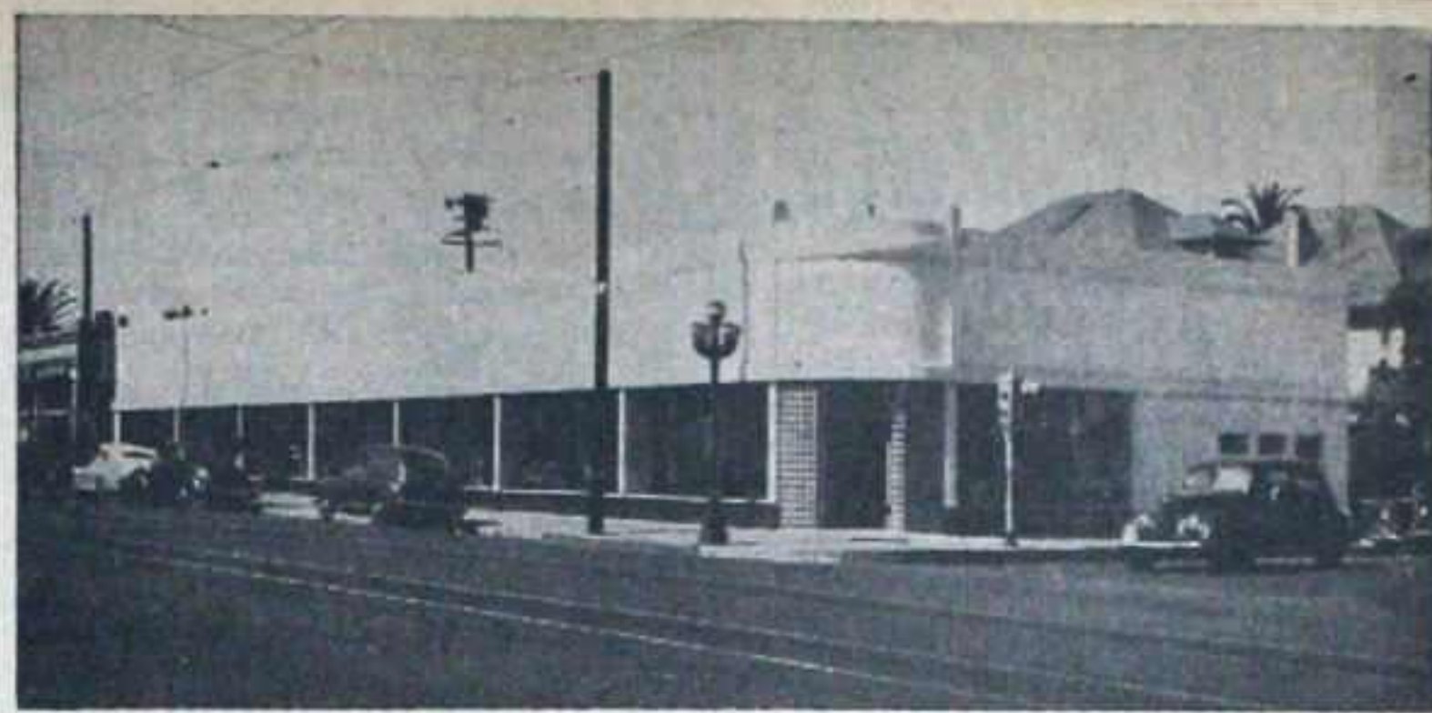
C. A. ROBINSON'S NEW LOS ANGELES HEADQUARTERS. Pictured above is the new home of C. A. Robinson, Los Angeles Buckley distributor. Five other tenants in the building are all associated with the industry and are all set for post-war trade. The building is located right in the heart of Coin Machine Row.
