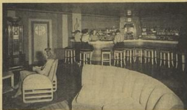
ROCKOLA'S SPECTRAVOX TONECOLUMN installed at the King of Clubs, swank spot outside of Green Bay, Wis. Badger Bay Company made the installation. (MR)
