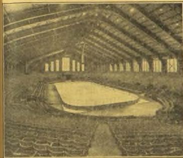
Interior of the Coliseum on Indiana State Fair grounds, Indianapolis. This magnificent auditorium normally seats 8,000, but for shows not requiring the arena the capacity can be increased to 11,000 by placing 3,000 chairs in the arena. There is not a post in the building, and every spectator has a full and unobstructed view.
