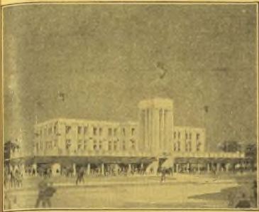
The 4-H Club building on the Minnesota State Fair grounds. Erected at a cost of more than half a million dollars, it is regarded as the finest structure of its type on the American continent. Measuring 357 by 150 feet, it is a three-story, fireproof monolithic concrete structure which provides an adequate setting for an impressive showing of the 2,000 of Minnesota's 50,000 4-H Club boys and girls who annually go to the fair.
