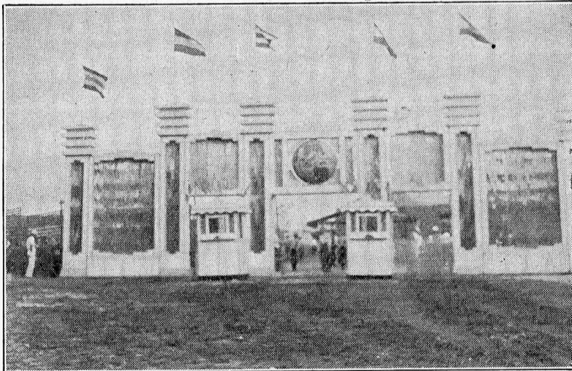
MUCH-TALKED-ABOUT ENTRANCE ARCH of Dodson's World's Fair Shows is 42 feet in height in the center and is 91 feet wide. Panels are in chromium with indirect lighting effects, while outside borders are covered with neon. Huge ball in center revolves continuously and carries neon wordage giving the title of the shows. The Dodsons have received much favorable comment, it is said, from prominent visiting managers regarding the arch.
