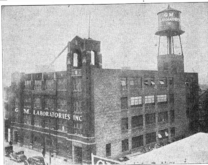
THE PLANT OF G-M LABORATORIES, INC., where the new games Shoot the Chutes and Soccer are now being made. Soccer was developed for British trade.
