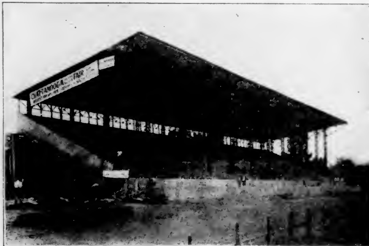
The Chattanooga Inter-State Fair, Chattanooga, Tenn., of which Joseph R. Curtis is secretary, has made a number of improvements since last year's fair. One of the most important was the erection of a new grand stand, which is pictured above. This stand has a seating capacity greater than the old, and is built of steel and concrete.
