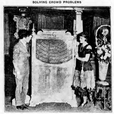
An important step in the solving of crowd problems in theaters has been taken thru the invention of vacant seat indicators which automatically show what seats are vacant. One of the latest of these devices is shown in the accompanying picture. It was placed in operation recently by Sid Grauman at the Grauman Million-Dollar Theater, Los Angeles. Mr. Grauman and Lois Wilson are shown watching the workings of the indicator.
