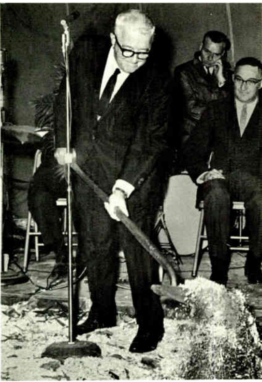
Judge Burton at the BMI groundbreaking
