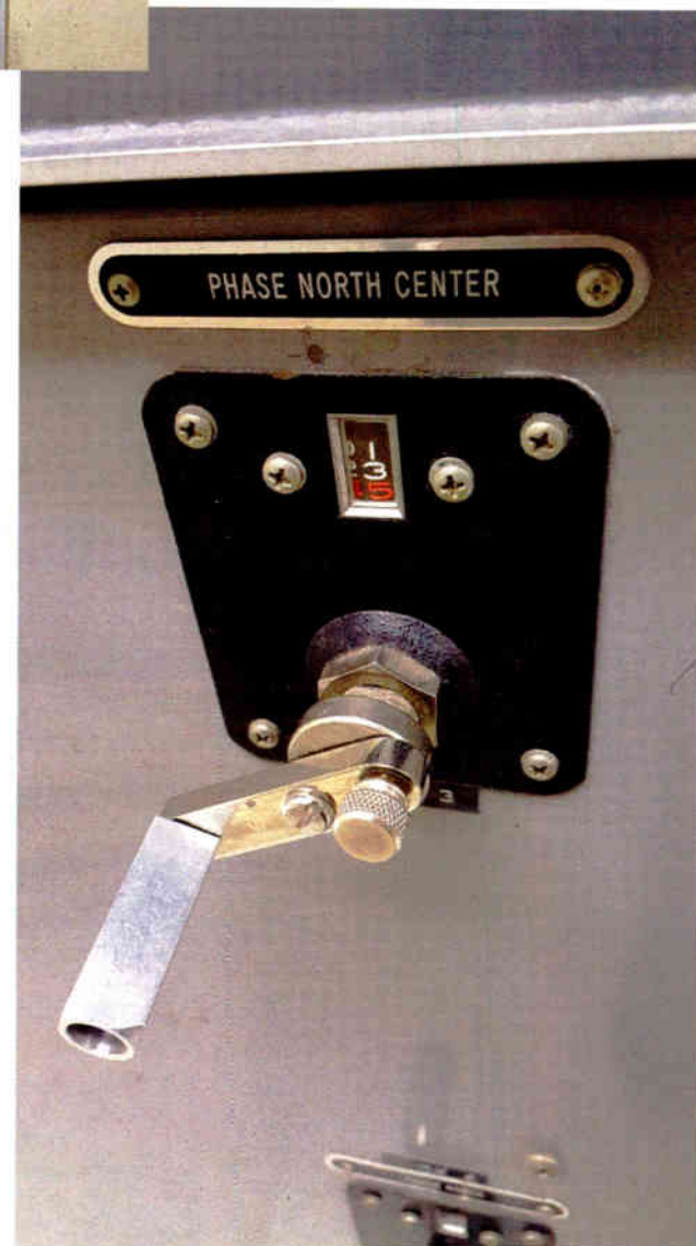
Fig. 2: Ensure tight set screws on phasor controls.
