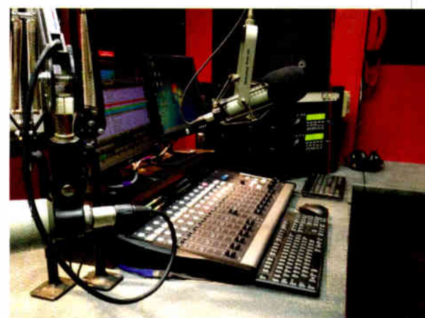
The finished studio.
