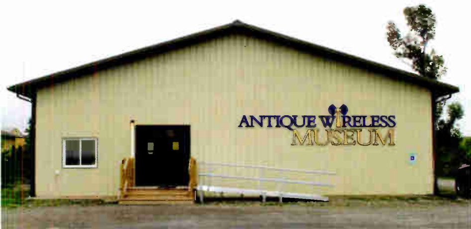
The Delano "big rig" now shares space in the AWA's new museum facility with a range of yesteryear's communications equipment.
