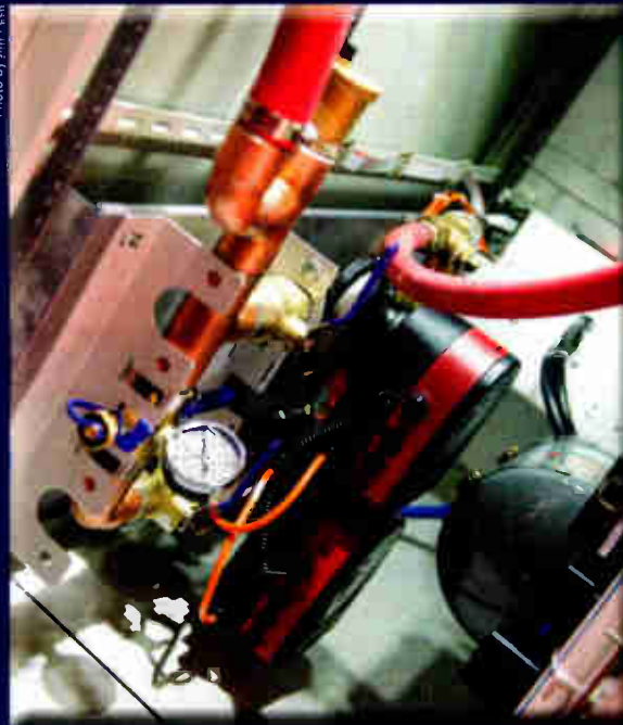
GatesAir introduced the FLX series of liquid-cooled transmitters. Shown are redundant circulating pumps, expansion tank and some plumbing. The 10 kW version can have pumps in the same rack as the transmitter proper. Heat exchanger assemblies, not shown, complete the loop. Liquid-cooled RF pallets are plug-and-play.
