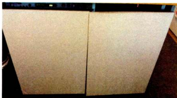
Fig. 1: Old and sagging doors are both unsightly and inefficient.
