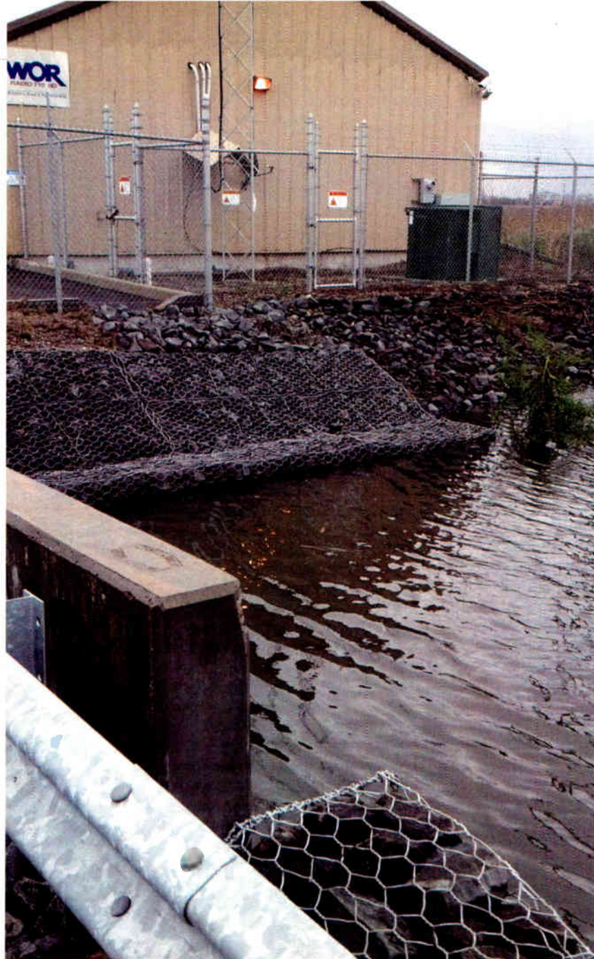
The water crowns at the front of the WOR transmitter building in Rutherford, N.J. Water is up to the top of its channel.
