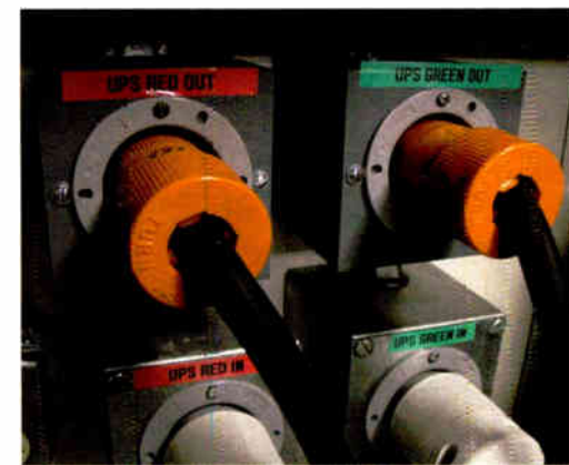
Fig. 2: Paul Shulins color codes the plugs for dual-UPS applications.
