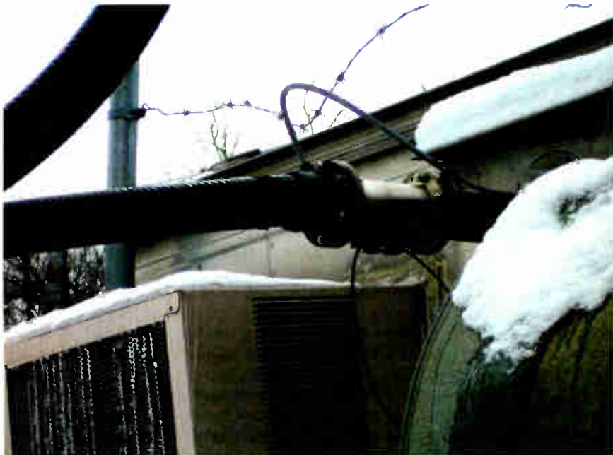
Fig. 2: Who knows what evil the elements will do to this directional coupler, mounted outside?
