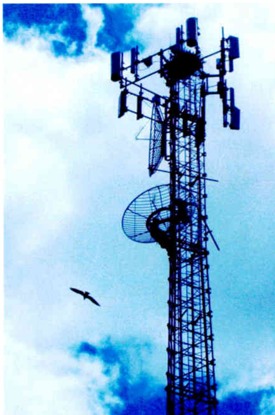
Fig. 1: As osprey watches as plastic Spike Strips are installed on STL dishes.
