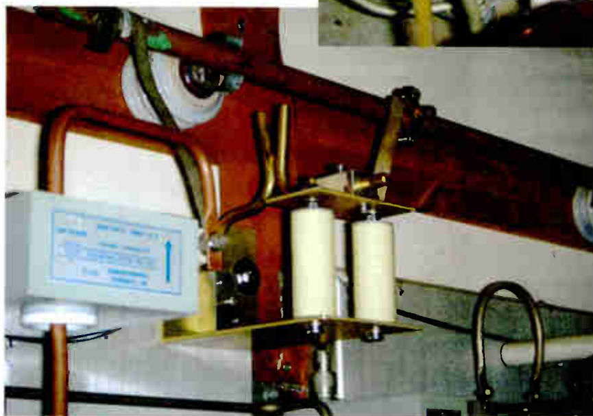
Fig. 1 (top): Trimming back the arced outer conductor stopped intermittent operation.
