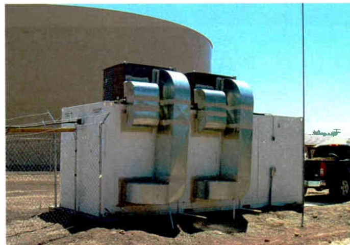
Fig. 6: After improvements, a transmitter building of which we can be proud.
