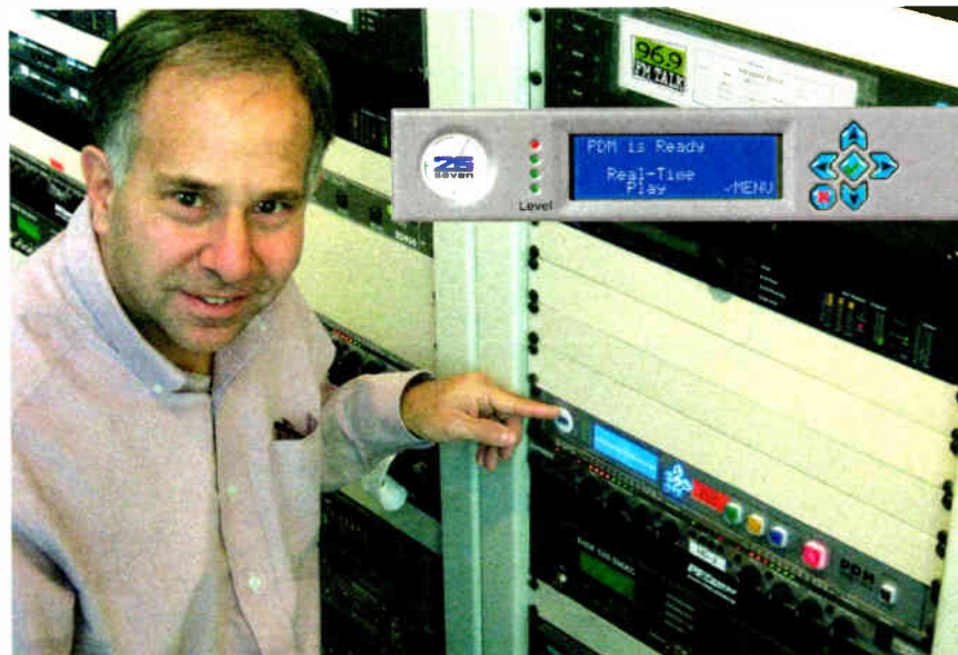
Paul Shulins points at the 25-Seven Systems Program Delay Manager in the rack at WTKK(FM).
