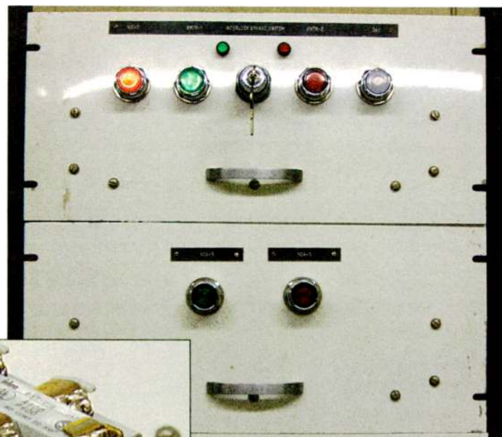
Fig. 2: Idec pushbuttons are used widely for phasor control panels.
