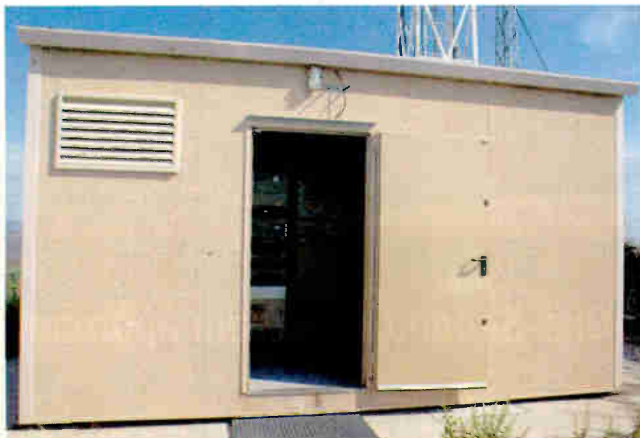
Fig. 1: A completed transmitter site building.
