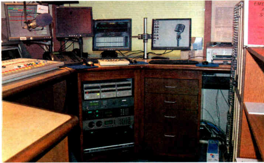
The Down-Under View of All the New Goodies
