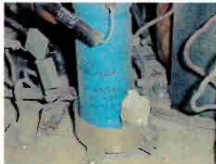
Fig. 3: A rock holds the capacitor stable.
