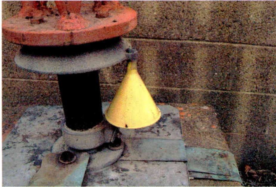
Fig. 1: An inverted funnel prevents spark gap shorting.
