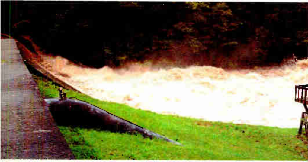
A 'penstock' at the base of the dam delivers water to the turbines in the powerhouse.
