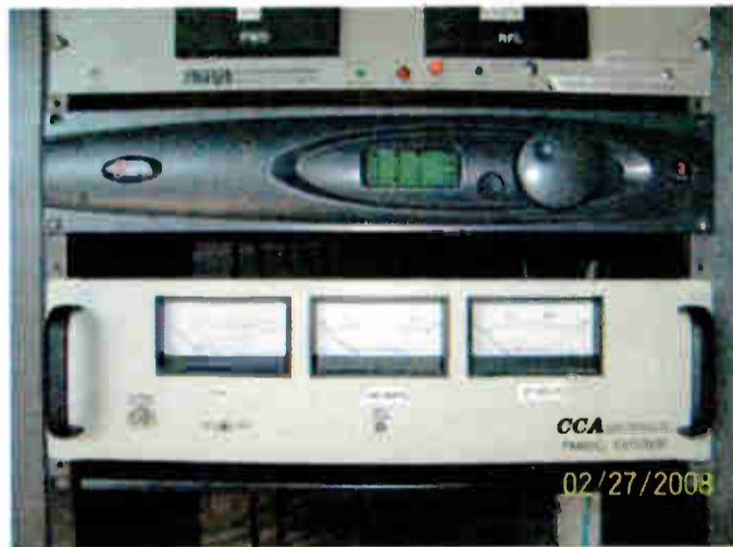
Fig. 2: Screwing the shelf below the heavy equipment provides support.
