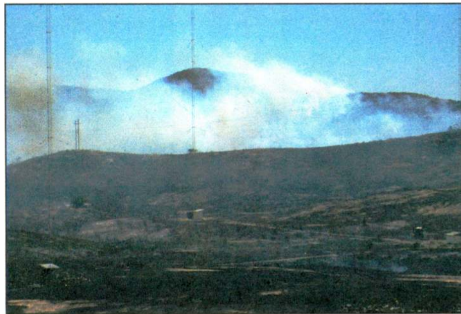
Fig. 1: The KBRT antenna field immediately after the fire moved through. Note that aggressive fire breaks left the antenna system intact.
