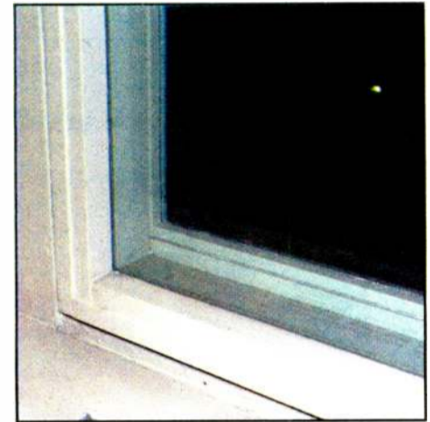
Fig. 4: This inside plate glass window reduced outside noise by over 60 dB.
