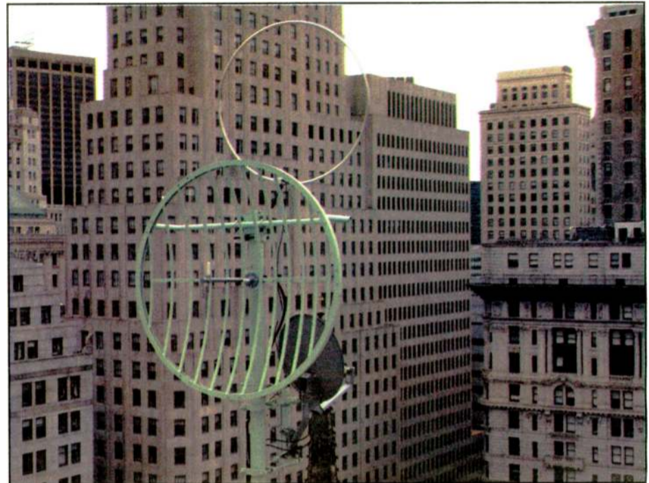
Fig. 7: The STL antenna, AM loop and DirecTV antenna mounted on the roof. The Mark grid dish is painted the same color as the building penthouse.
