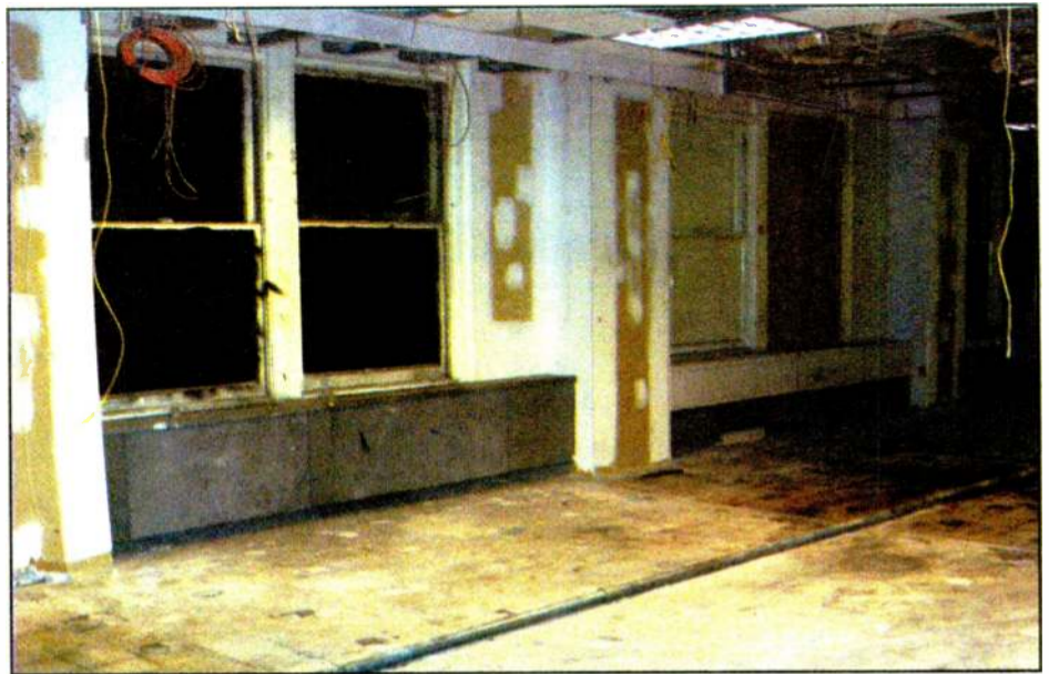
Fig. 3: This area would become the new master control room.
