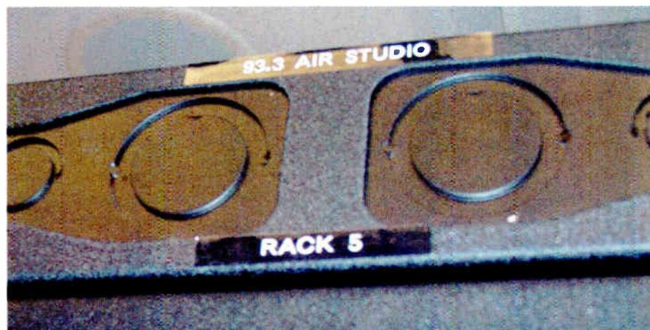
Fig. 2: Identify racks with the frequency, which, unlike call letters, is less likely to change.
