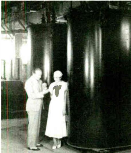
The 11-foot modulation transformers used in the WFLW 500,000 W plate-modulated transmitter. Image courtesy Charles Stinger, AWA.
