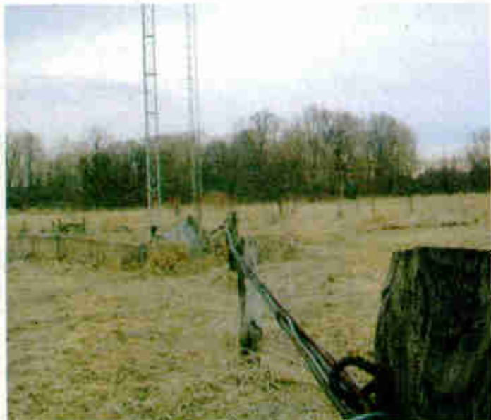
Fig. 1: View from the road of the tower and tilted ATU
