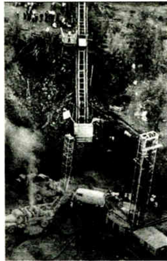
Aerial view of site with WMBT 'news cruiser' mobile unit at the center of the rescue operation. The WMBT unit remained for the duration of the rescue.
