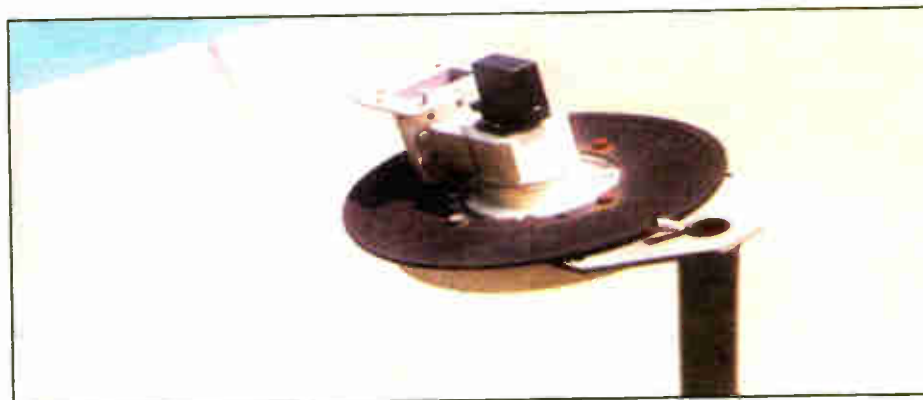
Fig. 5: Inspect satellite feedhorns and cap openings.
