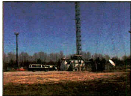
Fig. 1: Even a temporary tower can wreak havoc with an AM directional.
