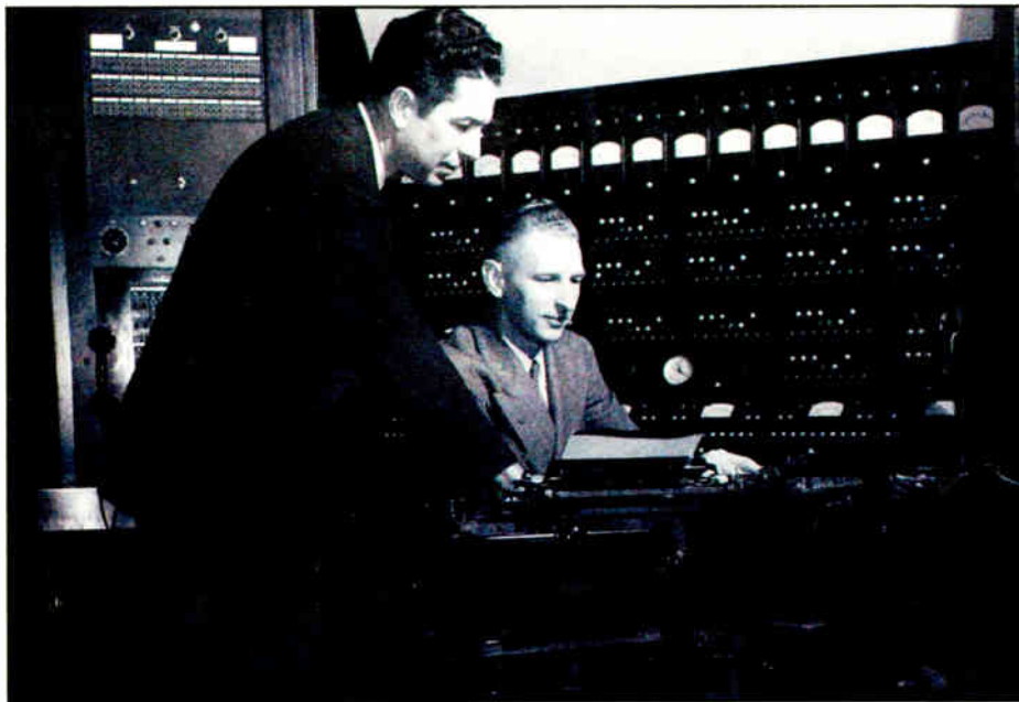
Master Control Room at NBC's Radio City in San Francisco, December, 1944. Standing: George Greaves, engineer-in-charge of NBC San Francisco. Seated: Lee Kolm, control room supervisor. The operator determined which studio program was fed to which broadcast phone line on the network. Fourteen circuits could be fed simultaneously. All programs fed to KPO, KGO and the two networks originated here. Audio patch panels could be used to substitute a failed studio amplifier in case of emergency. A telegraph sounder on the desk was used to communicate with the KPO transmitter in Belmont.
