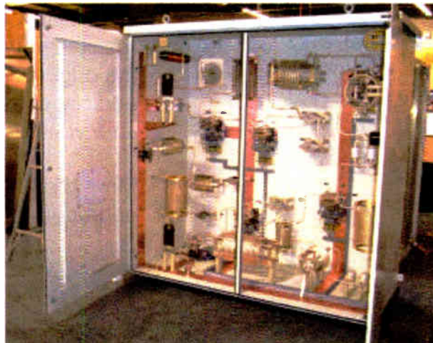
DIRECTIONAL ARRAY ANTENNA TUNING UNIT GAITHERSBURG, MD
