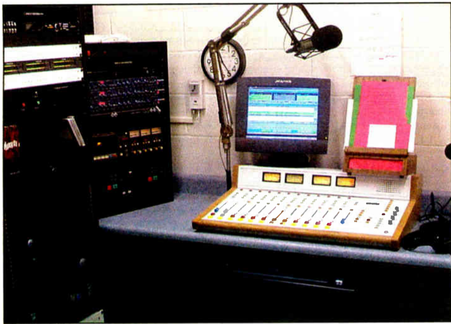
The Equipment at the Nearly Complete WNHS(LP) Studio
