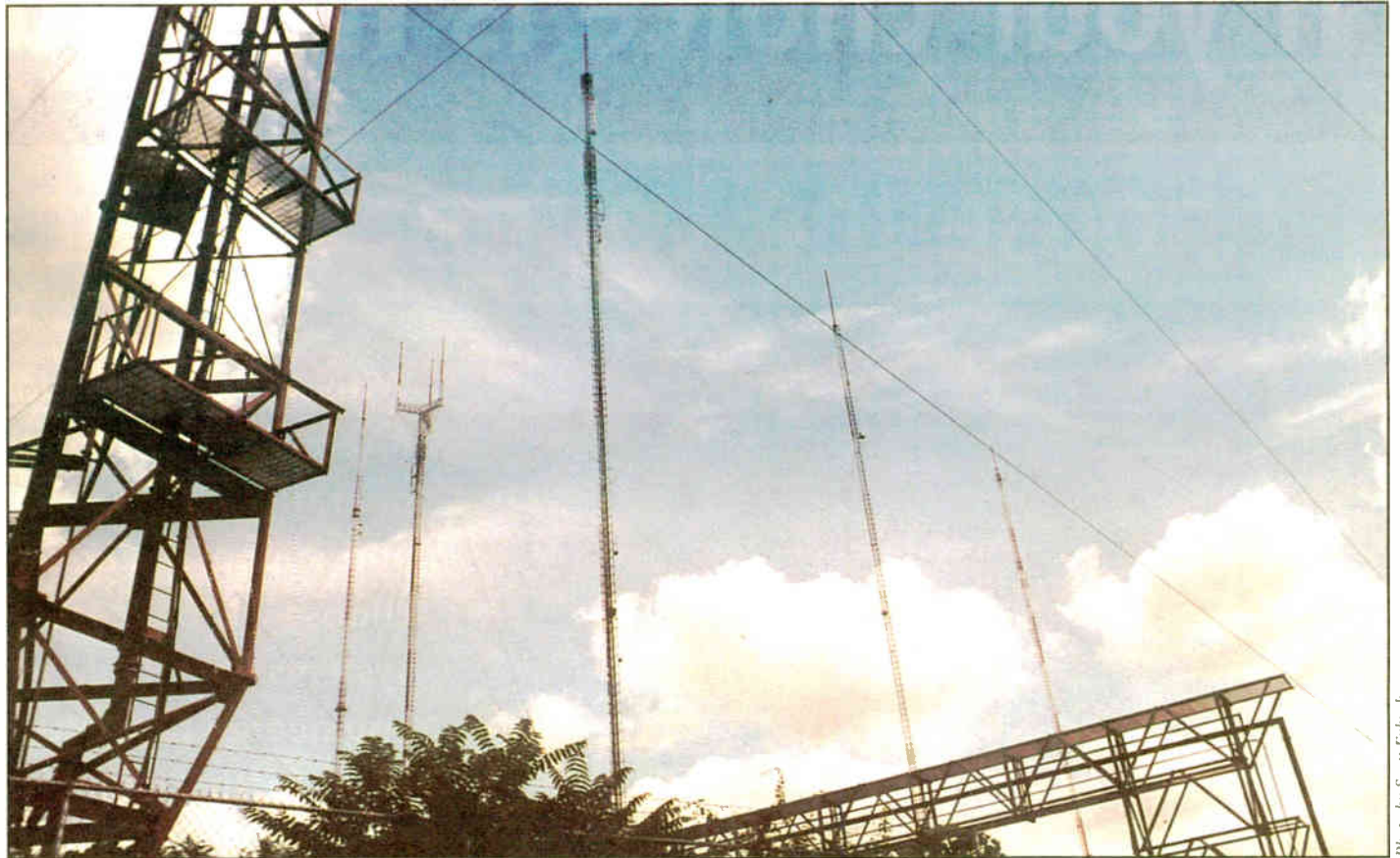
From left: WGTW(TV); the old WCAU(TV) tower; the new Philadelphia digital TV tower; and the Banks, Fox and Gross Towers.
