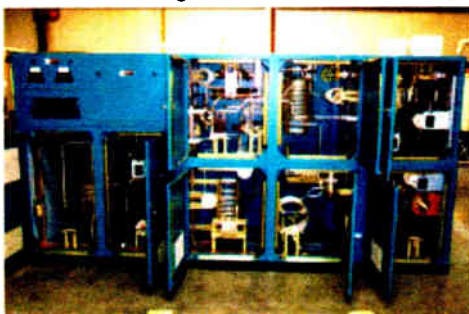
THREE TOWER AM 50kW NDA-D / DA-N DIRECTIONAL ANTENNA SYSTEM ST PAUL, MINN.
