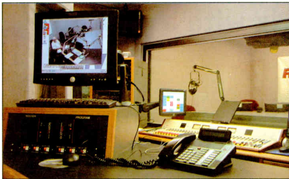
The Studio B talent area looks into the control room; the news booth is in the rear. On-air programming originates from both Studios A and B.
