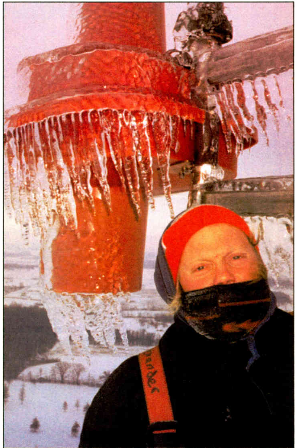
Antenna systems must be inspected to assure proper operation, particularly when the weather turns nasty. This three-bay Shively 6813 serves Richmond, Ohio.
