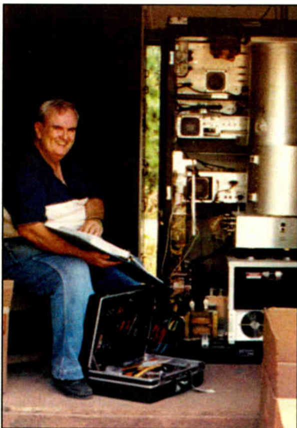
Clayton Caughill is shown installing a Broadcast Electronics FM5B FM transmitter for Radio1 in Tahiti, October 1993
