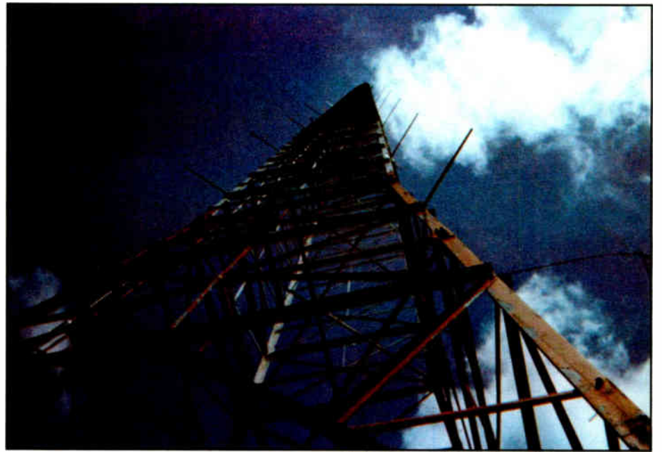
This skirted DA tower is part of the three-stick array of KKPZ(AM) on Mt. Scott in Portland, Ore. It supports an FM antenna for KUPL(FM).
