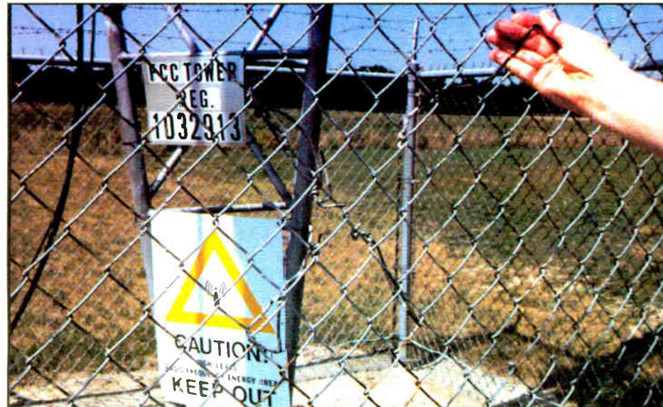
Figure 1: Affix signs on the tower to thwart thieves.
