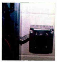
Figure 2: A spare 220VAC outlet box will speed installation of an emergency low-power transmitter.
