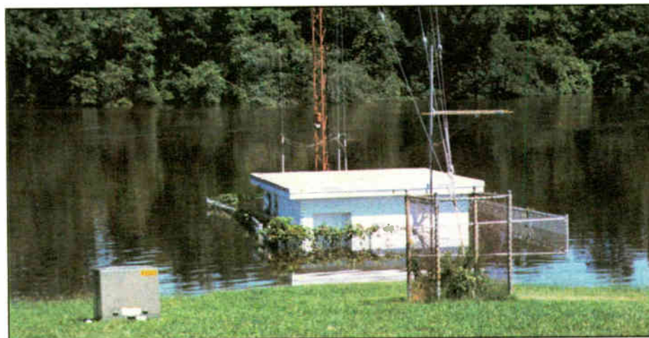
WOOW's transmitter building was submerged by floodwaters.
