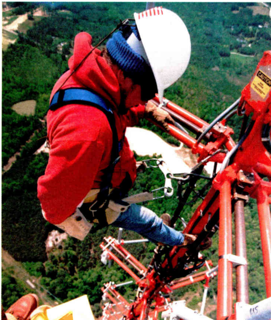
Figure 3: At 1,200 feet, the remaining antenna elements are installed.
