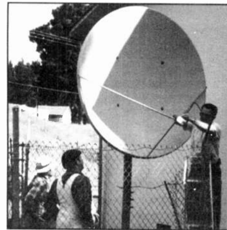
KLVM(FM) engineers install the station's digital audio network uplink.
