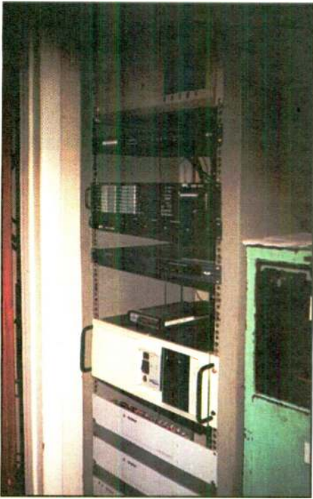
One rack holds satellite receivers, EAS Decoder/Receiver, digital storage computer and Gentner remote control VRC 2000.
