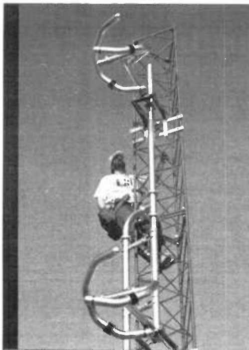
ERI, SHPX series FM Antenna and \lambda Mounting System
