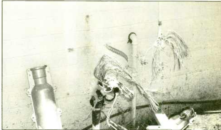
Thieves left a massive splice job for the phone company.
