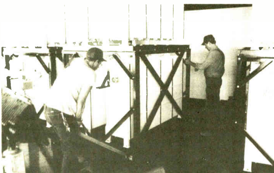
Workers ease one of the combiner elements into place (left), fit the elements into a rack (center), and start the process over with another element (right).
