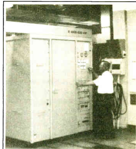
The AEG Telefunken S4005 is one of the four 500 kW transmitters purchased by the VOA for evaluation. Shown at right is John Moss, station manager.
