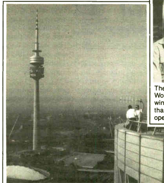
The roof of the BMW car factory becomes the site of a repeater antenna. The Olympic tower (left) stands guard.
