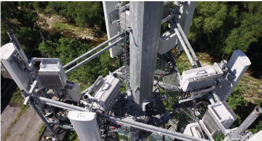
Detailed information can be captured where an unobstructed view is possible.
